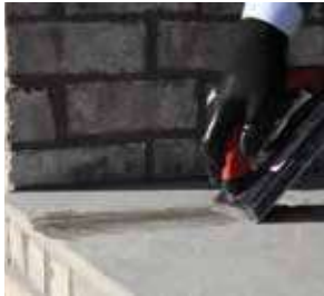
PIC 1. Fill joint with grout.
